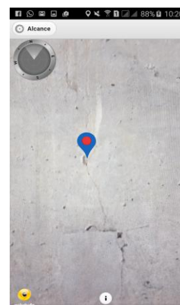
Figure 3: Dam Cracks Information Prototype screen.
